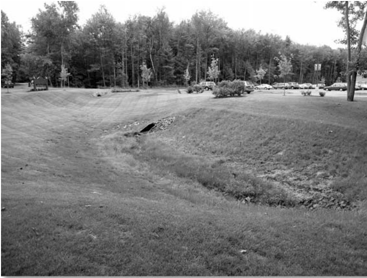
This infiltration basin handles the stormwater from a large parking lot, catching pollutants as the water seeps into the soil. This practice replenishes local groundwater, rather than allowing stormwater to be lost. Integrated into the landscaping, the basin adds to the appeal of the property.
