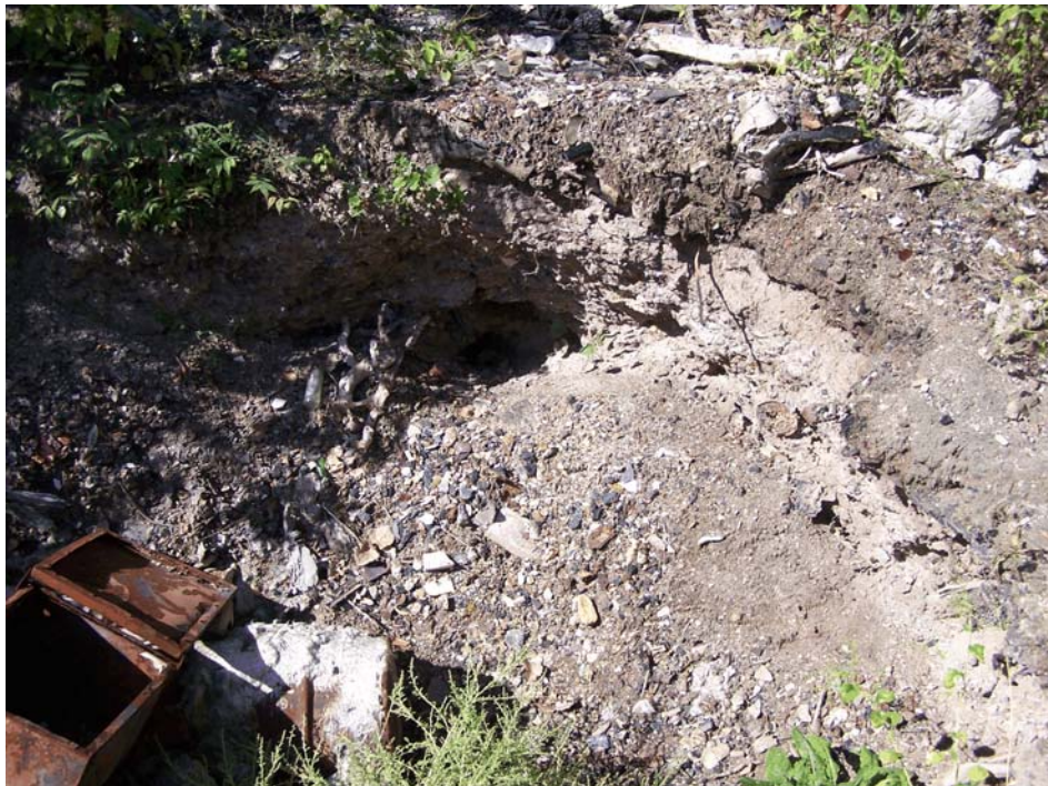
Figure 6-12. Photograph of a pit excavated into the ash by individuals apparently scavenging for antique bottles and other items. View looking west. Photograph taken by Glenn May on October 1, 2007.
