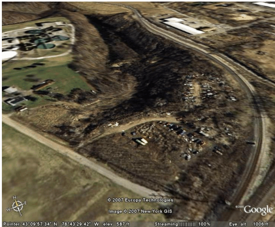
Figure 6-2. Aerial photograph of the Old Upper Mountain Road Site showing the steep slopes of the ravine, the junk automobiles and site roadways. View looking northeast. Photograph downloaded from Google Earth on May 22, 2007.
