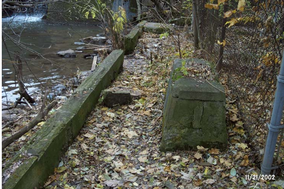
Figure 2-1. Photograph of the fenced containment structure that may have housed transformers and/or capacitors containing PCB oil. The Clinton Street dam is in the background, while Eighteenmile Creek is to the left. Photograph taken by Paul Dicky on November 21, 2002.
