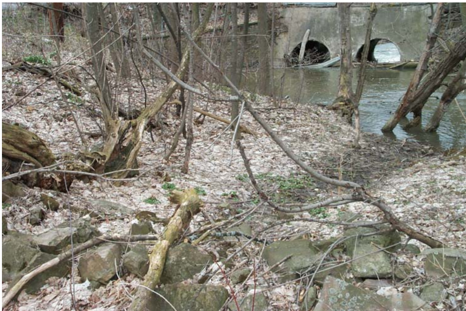
Figure 5-6. Photograph of the natural drainage swale from the side yard of 143 Water Street to Eighteenmile Creek. The cross-culverts beneath William Street can be observed in the background. Note the debris partially blocking these culverts. Photograph taken by Paul Dicky on April 16, 2002.
