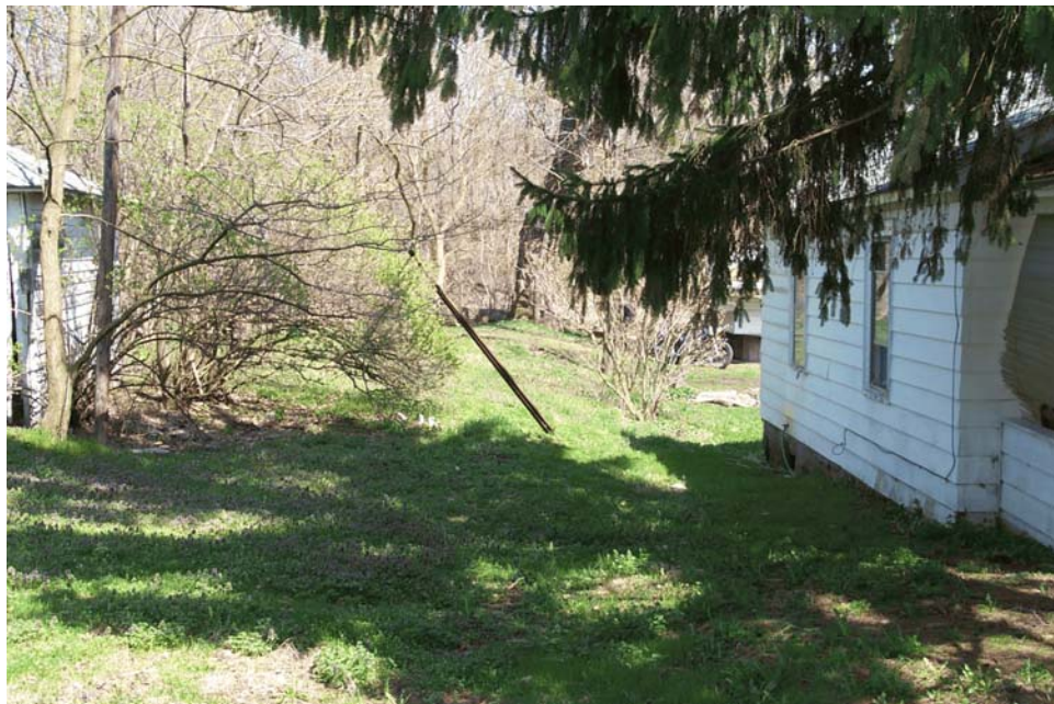
Figure 5-4. Photograph of the property line between 131 and 127 Water Street. The elevation difference (about 3 feet) delineates the extent of ash-cinder fill at the 143 and 131 Water Street properties. Photograph taken by Paul Dicky on April 16, 2002.
