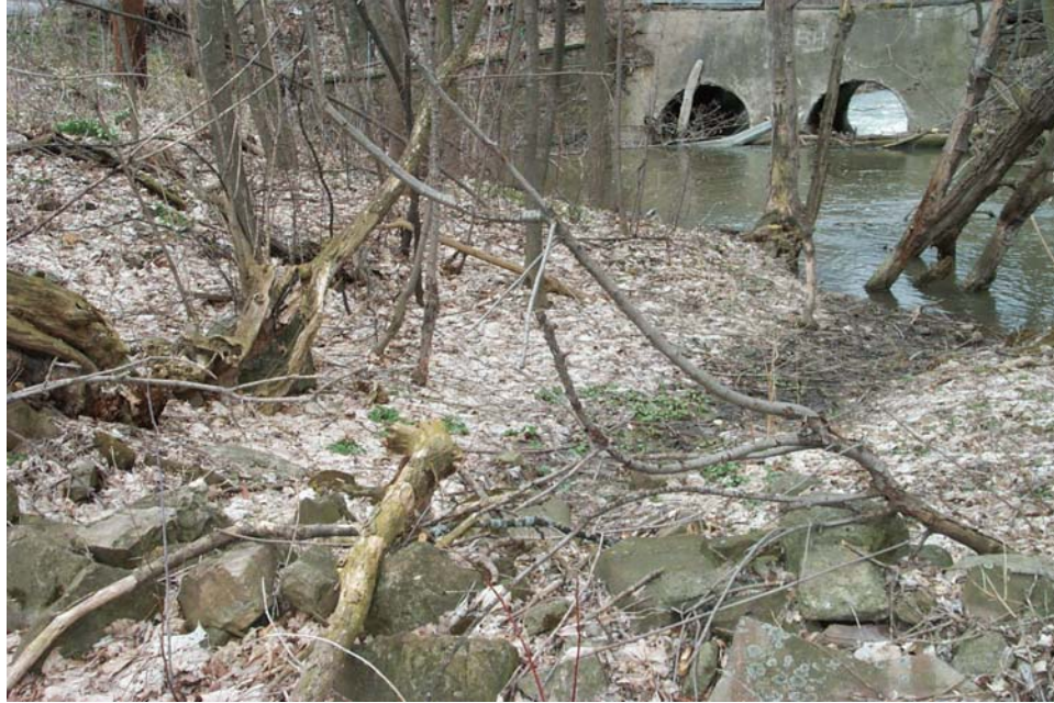
Figure 5-5. Photograph of the natural drainage swale from the side yard of 143 Water Street to Eighteenmile Creek. The cross-culverts beneath William Street can be observed in the background. Note the debris partially blocking these culverts. Photograph taken by Paul Dicky on April 16, 2002.
