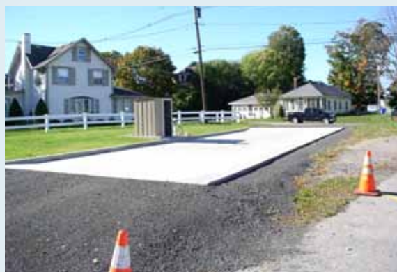
Concrete boat wash pad at Olcott with catch basin drain.
