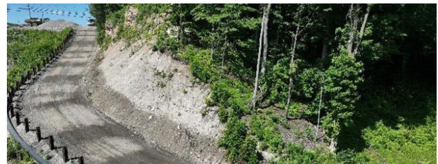
Construction access roadway with pile reinforcement
