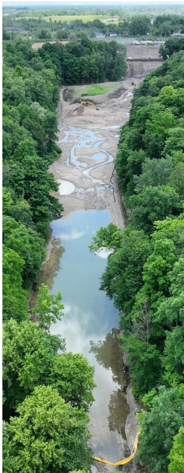
Restoration Progress, Summer 2024
