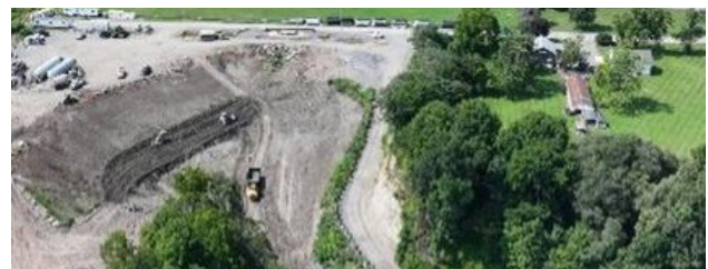
Sediment amendment and consolidation on steep slope
