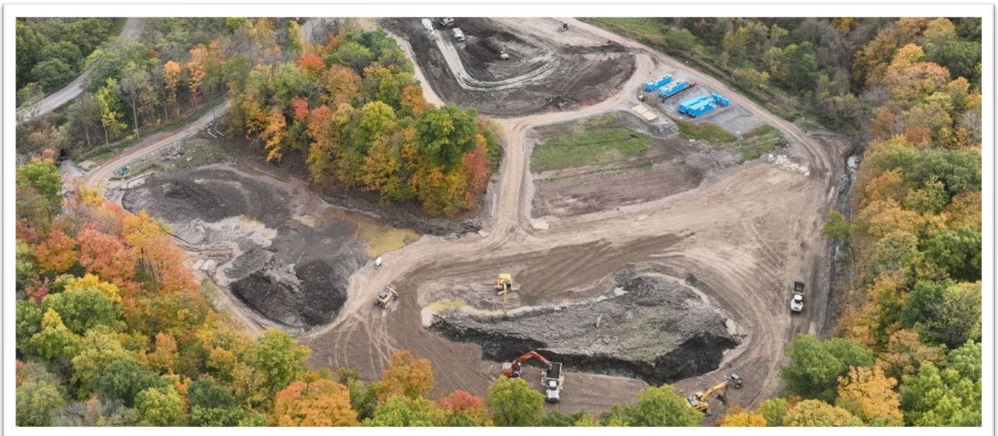
Sediment excavation, processing, and backfilling downstream Gulf Creek, October 2023
