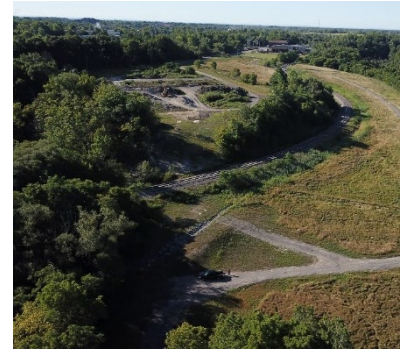
Restored surfaces along completed sewer alignment, access road left in place for future use
