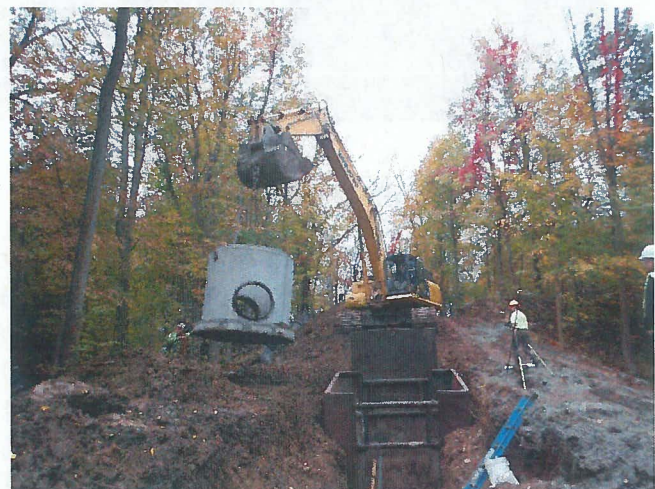
Installation of sewer manholes.
