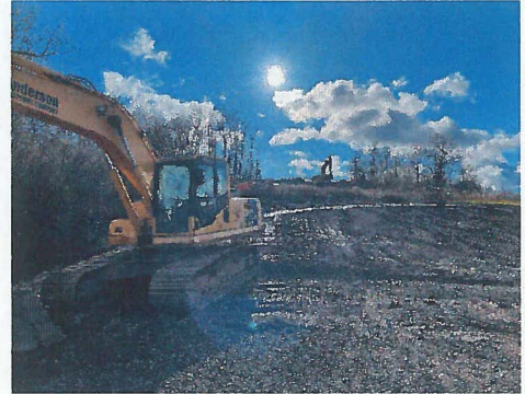
Restored surfaces post-installation
