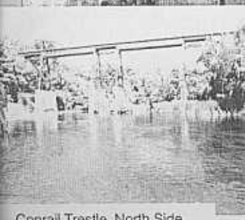
Conrail Trestle, North Side
